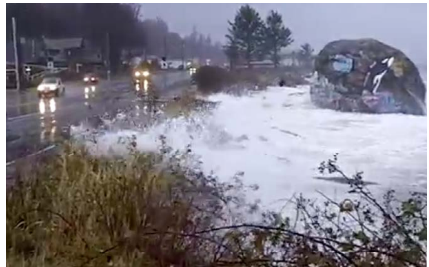
Waves at edge of highway during storm in November 2011
